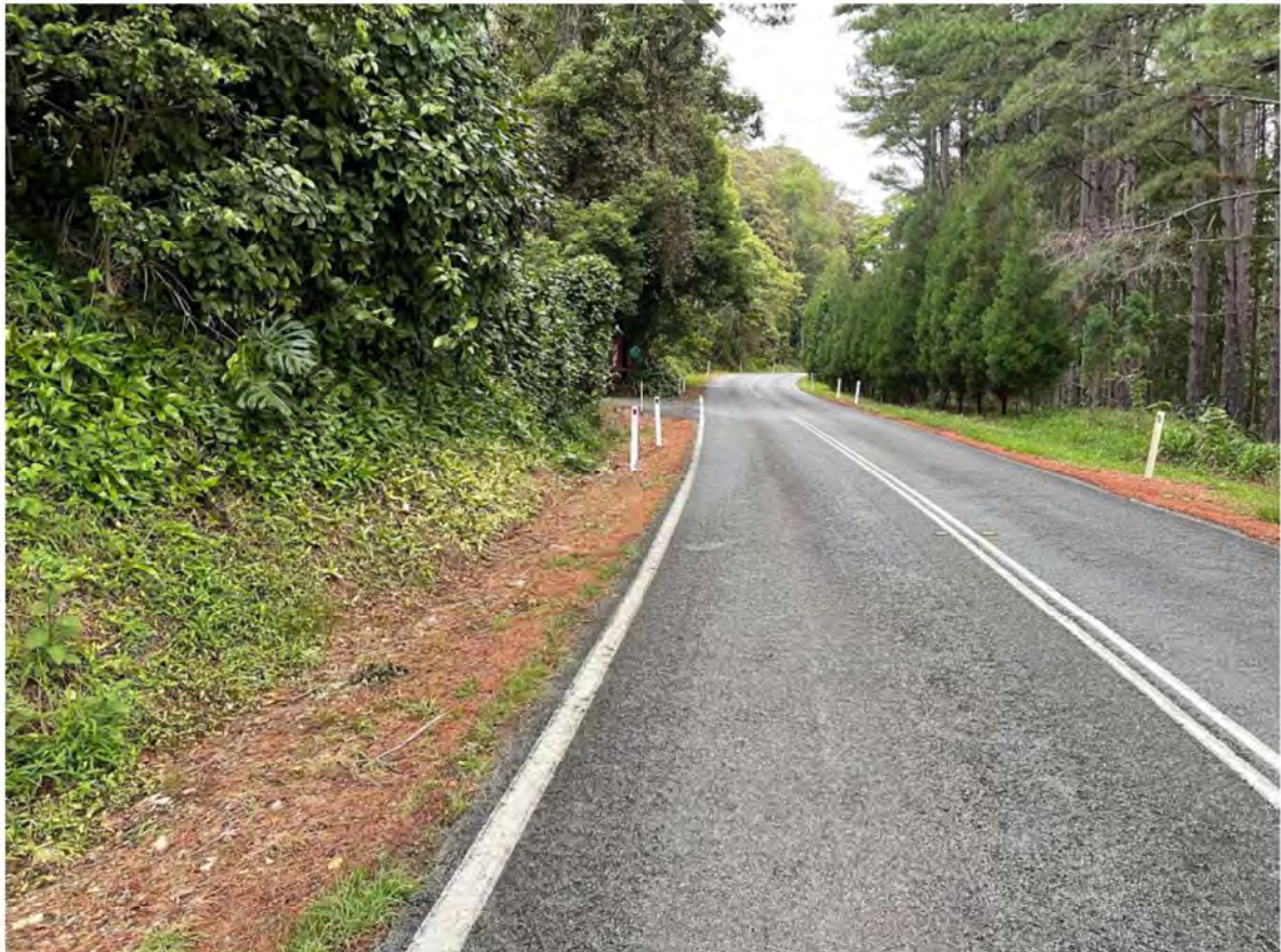
View from proposed shared drive looking south to Border Gate with NSW. Very clear visibility.
