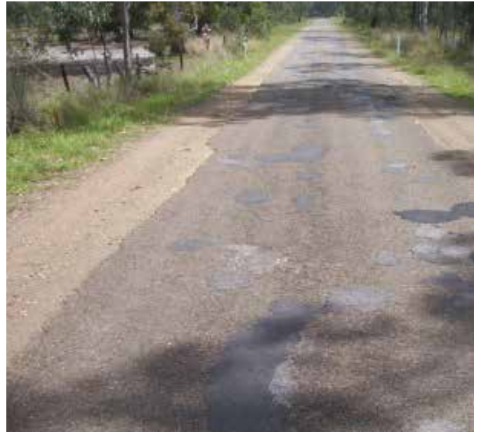
Mt Larcom Bracewell Road before
