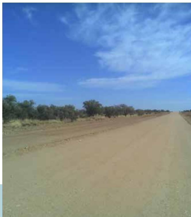
Donohue highway after resheeting
