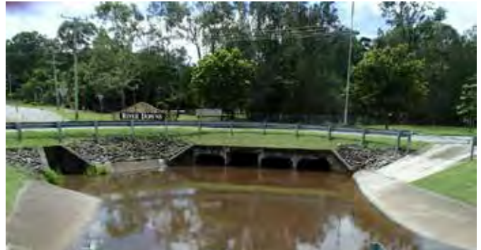
Helensvale Road before
