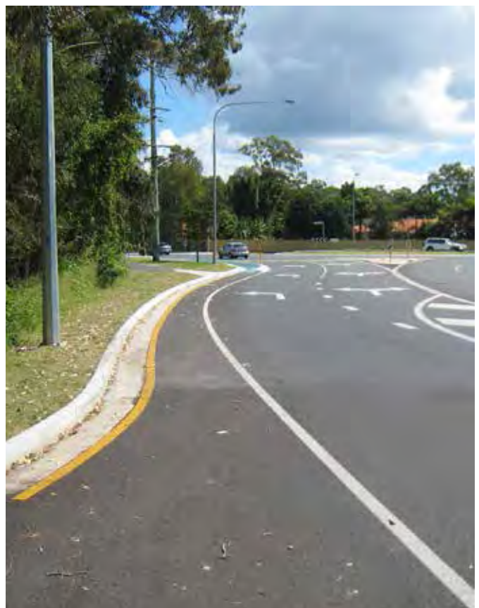
Helensvale Road after the upgrade
