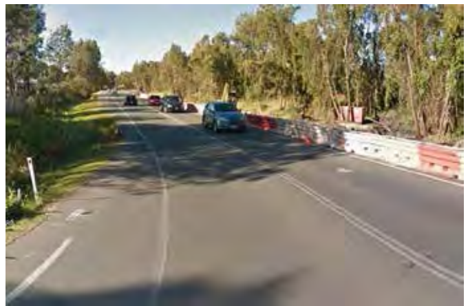
Helensvale Road during the upgrade
