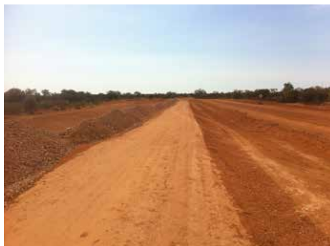
Donohue highway during resheeting
