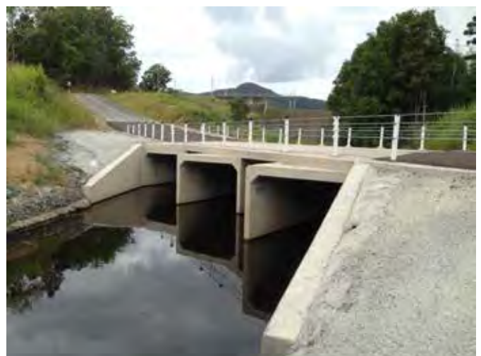
Gears Bridge after the project
