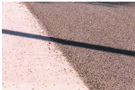
Figure 6.3.3.3(d) – Immediately after placing aggregate for second spray run
