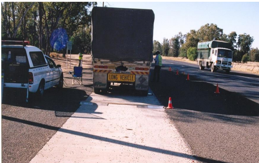
Figure 6.2.1.2.1(b) – Completed screening area with adjacent seal (prior to linemarking)
