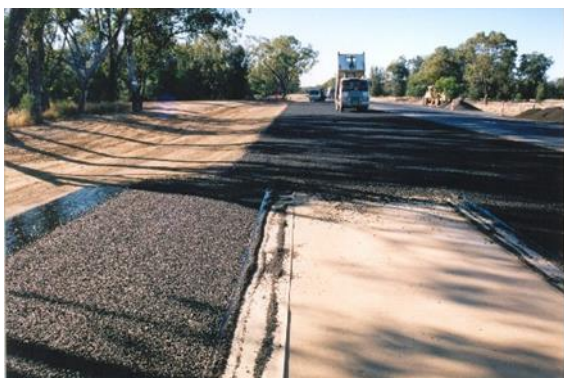
Figure 6.3.3.3(c) – Immediately after placing paper for second spray run
