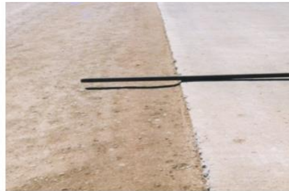
Figure 6.2.1.2.2(b) – Pad and pavement level
