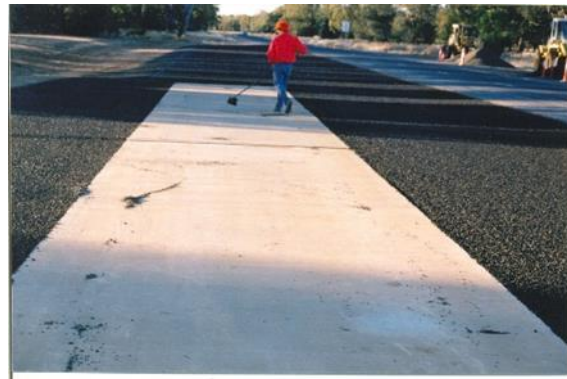
Figure 6.3.3.3(d) – Immediately after placing aggregate for second spray run
