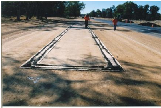
Figure 6.3.3.3(c) – Immediately after placing paper for second spray run
