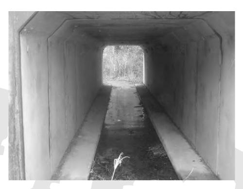
Plate 1. Culvert with dry ledges
