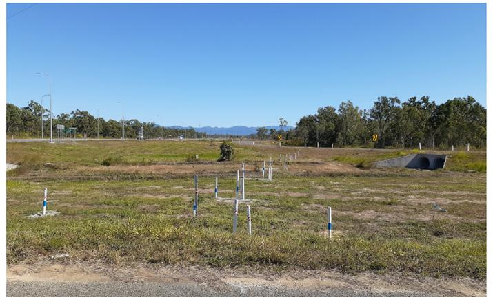
Colour coded pipes identify underground utilities.
