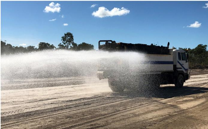
15,000 litre water trucks help to mitigate dust impacts during construction works.
