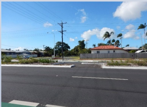
Image: Completed cycle refuge crossing (Source Arup 2016)
