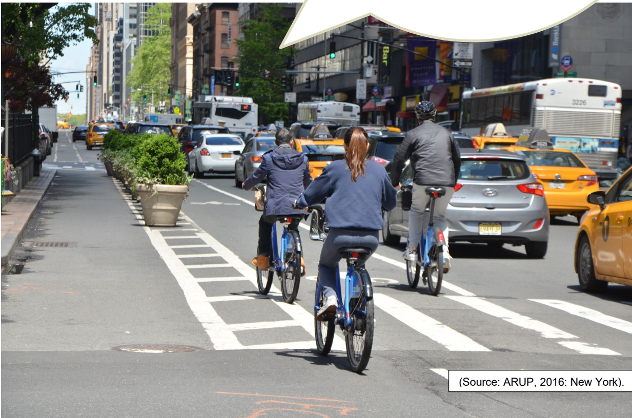
Figure 13 Innovative treatment – footpath widening and one-way protected cycle track, Broadway, New York City, NY
