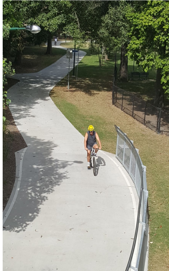
Figure 4 Widening on cycleway provides offset to fencing
